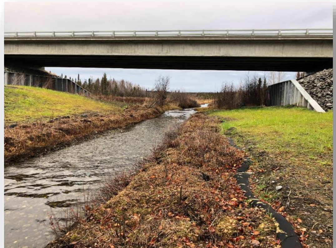
NEW 104' X 18' bridge
