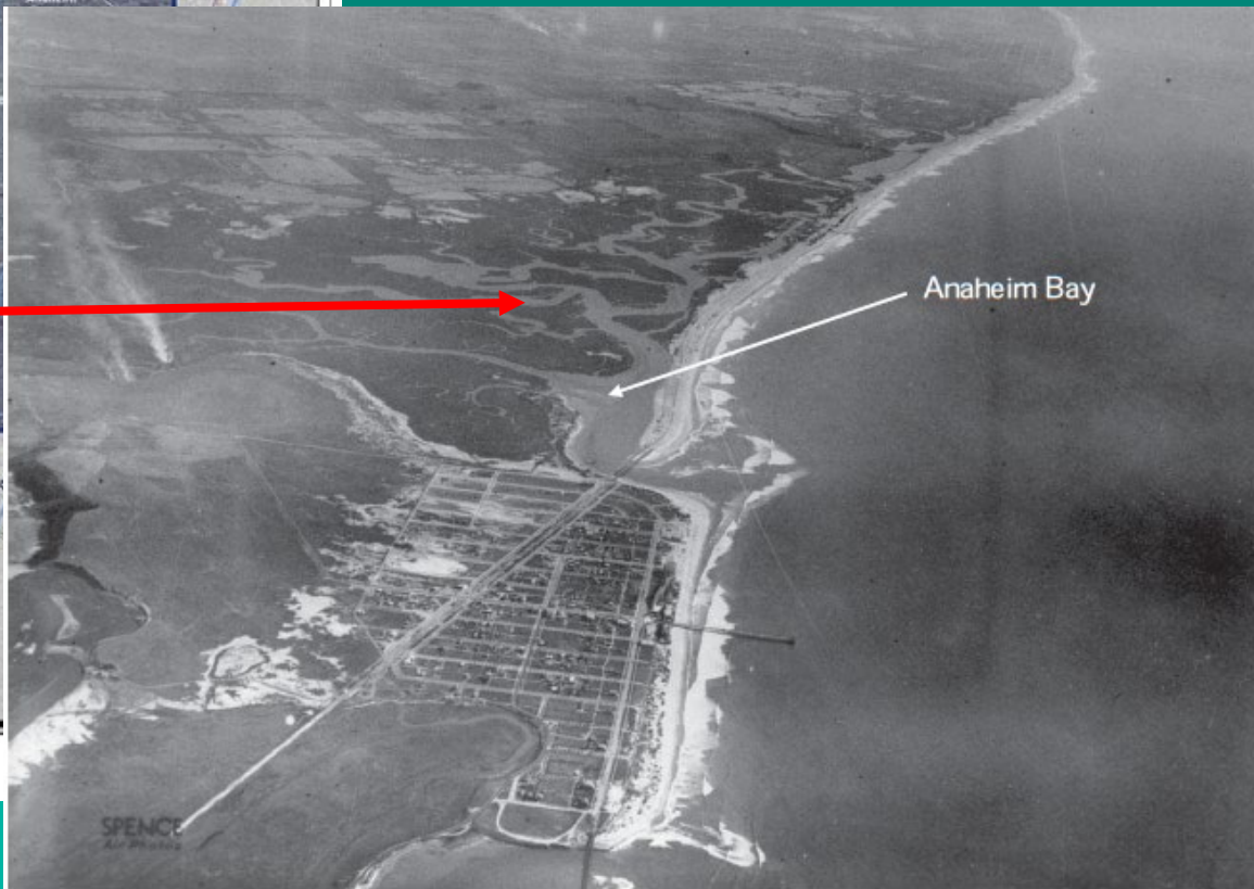
Figure 4-4. Aerial View of Anaheim Bay and Salt Marsh Complex in 1922
