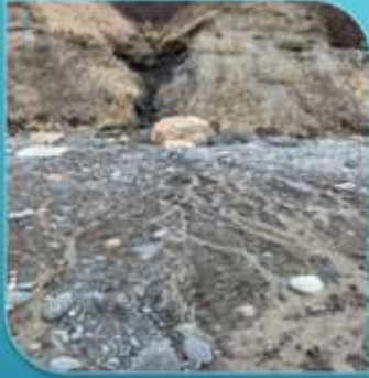
Storm water erodes channels and deposits on beach
